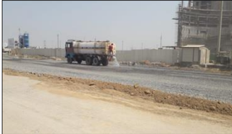
Water Sprinkling on Roads
